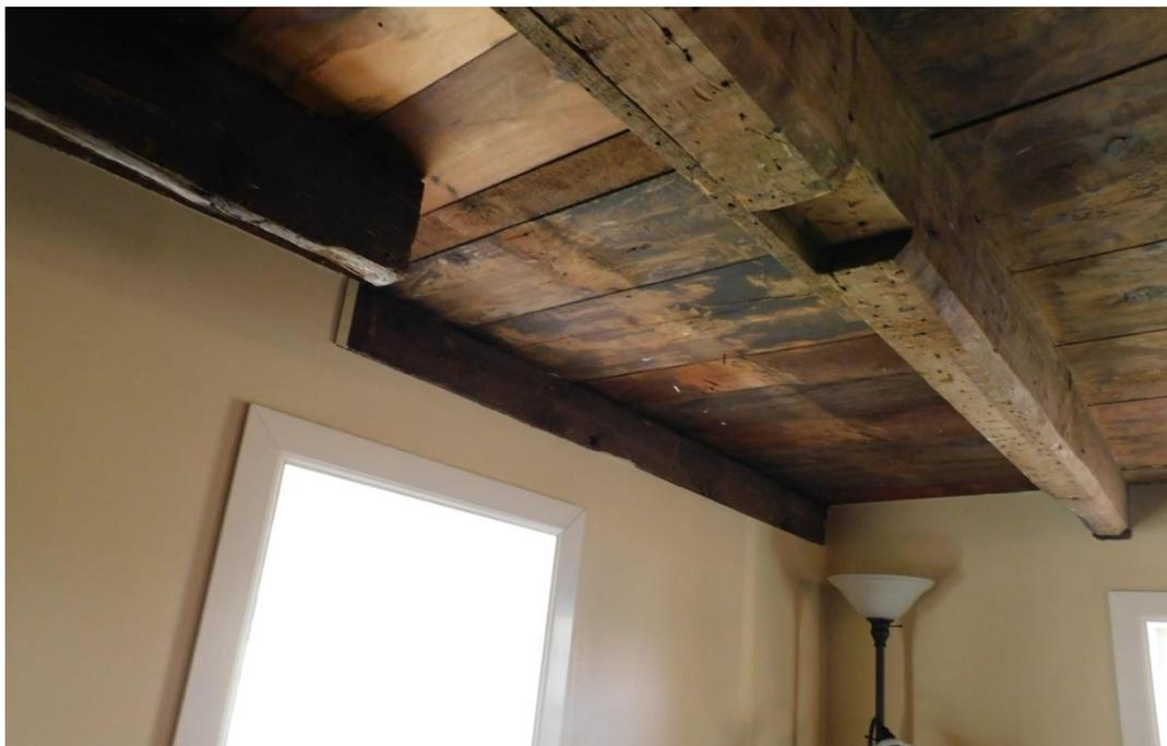
East end of kitchen wing showing original location of fireplace and floor joists
